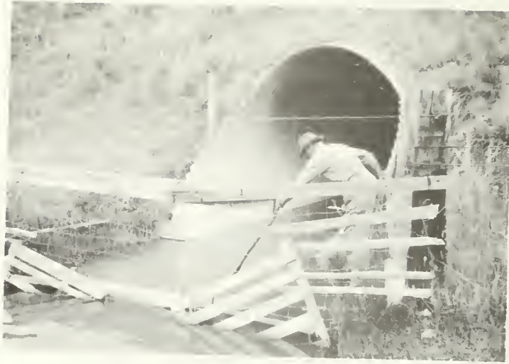
NORTH ENTRANCE High Water
